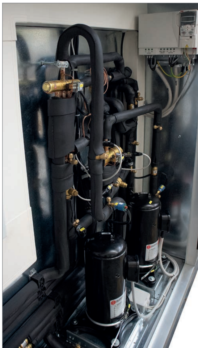
REFRIGERATION CIRCUIT
