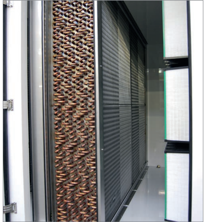
SPECIAL TREATMENT COILS
