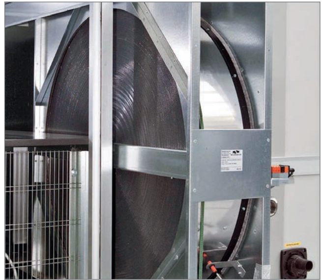
ROTARY HEAT WHEEL EXCHANGER
