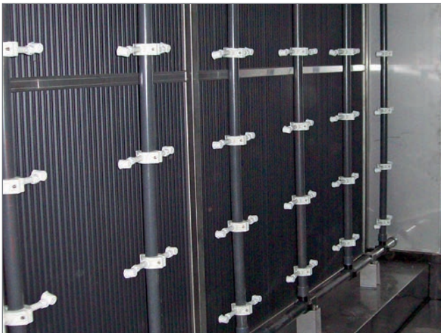
NOZZLES HUMIDIFICATION
