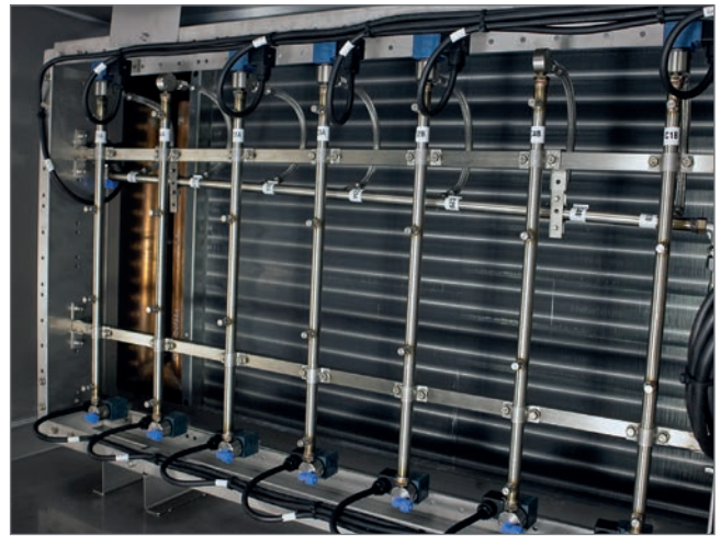
HUMIDIFICATION WITH PRESSURIZED WATER
