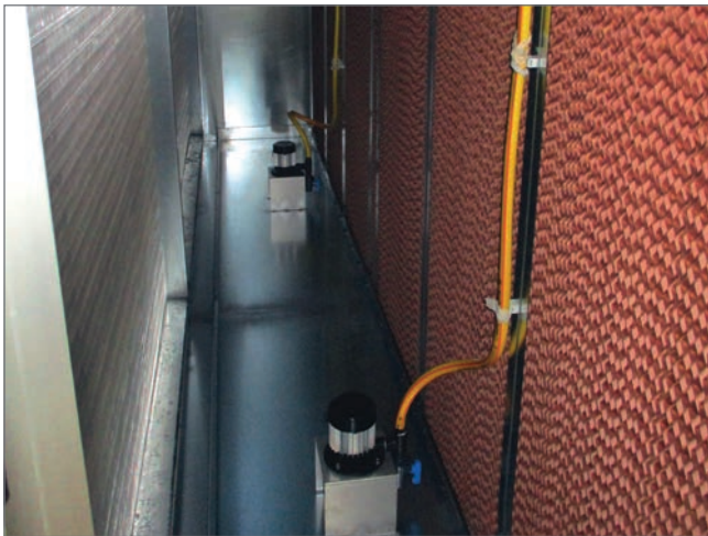
HONEYCOMB HUMIDIFICATION
